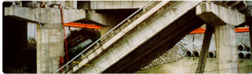
Collapse of Shi-wei Bridge, 1999 Chi-Chi Taiwan earthquake (Photograph by Ian G. Buckle, MCEER)
